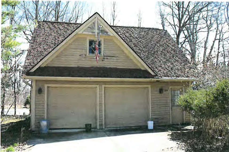
High 320, Garage_Looking East
