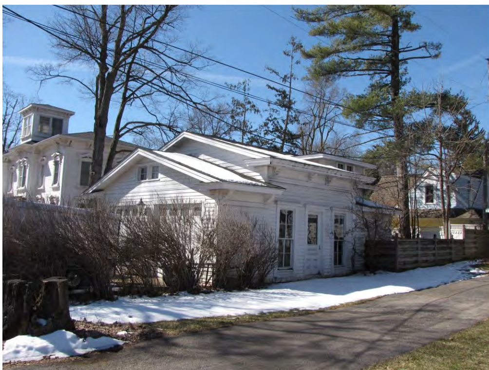
Dunlap West 404, Garage_Looking Southwest
