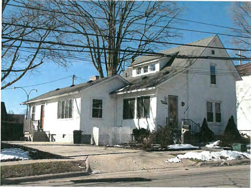
Randolph 113_Looking Southwest
