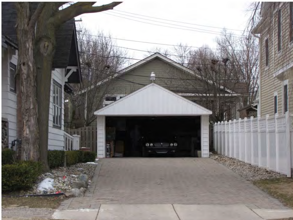
Wing North 111, Garage_Looking West
