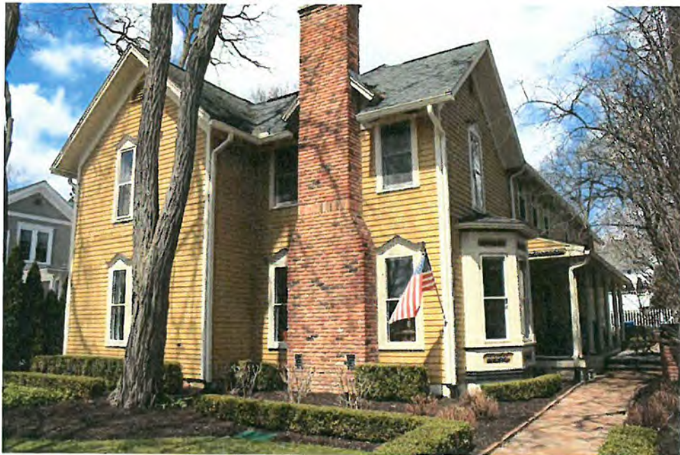
Main West 536_Looking Northwest
