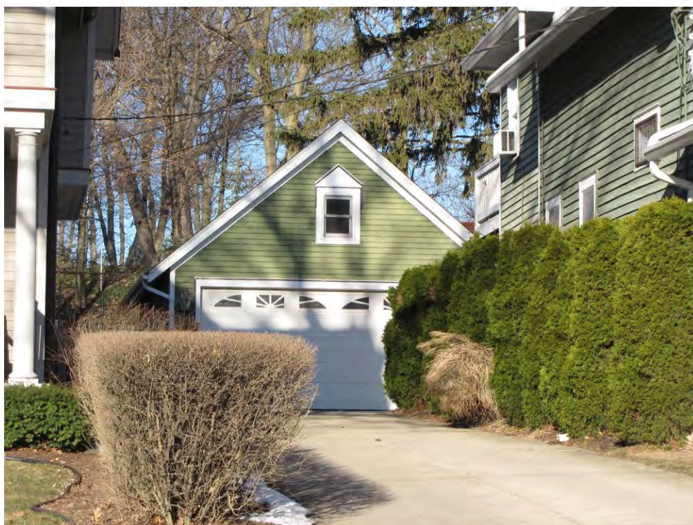
Rogers North 359, Garage_Looking West
