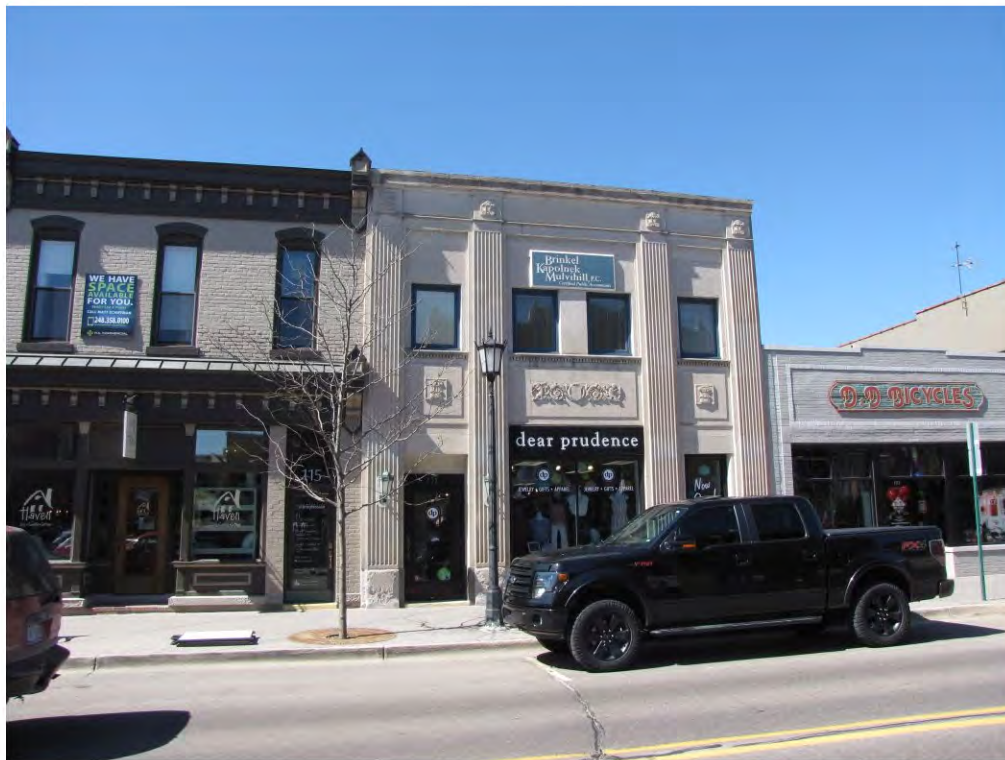
Center North 119_Looking Northeast
