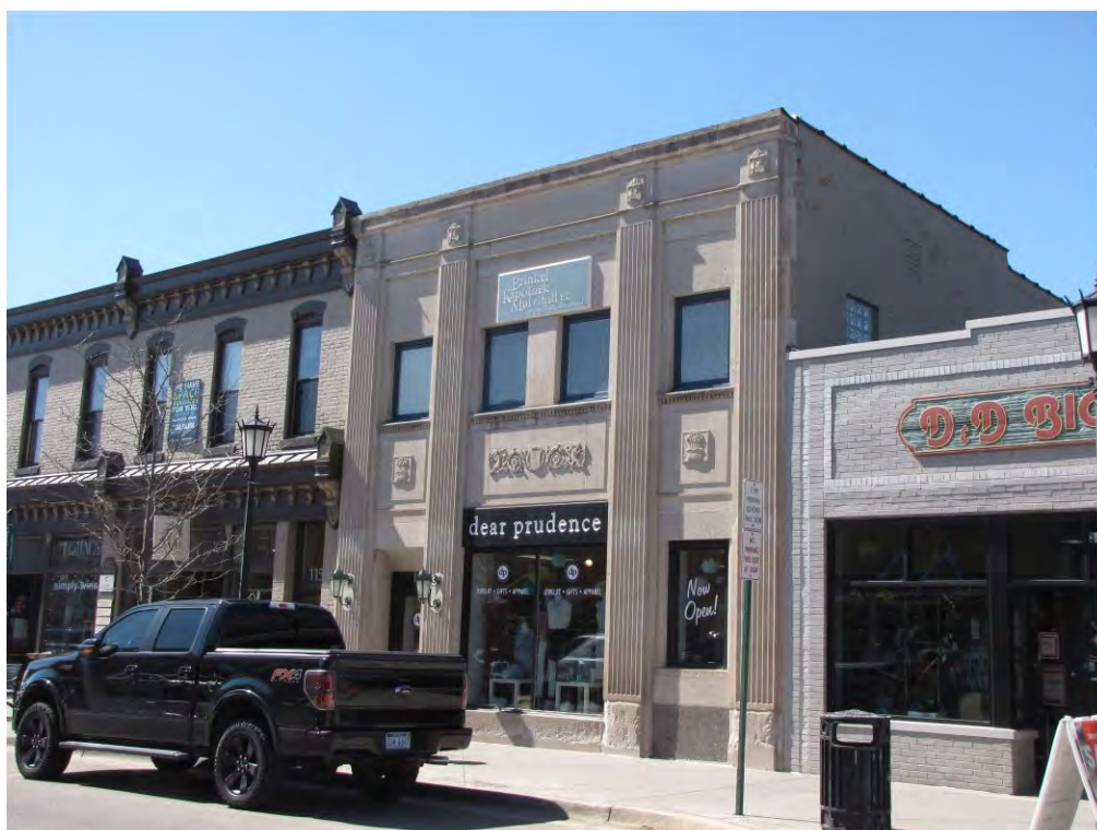
Center North 119_Looking Southwest
