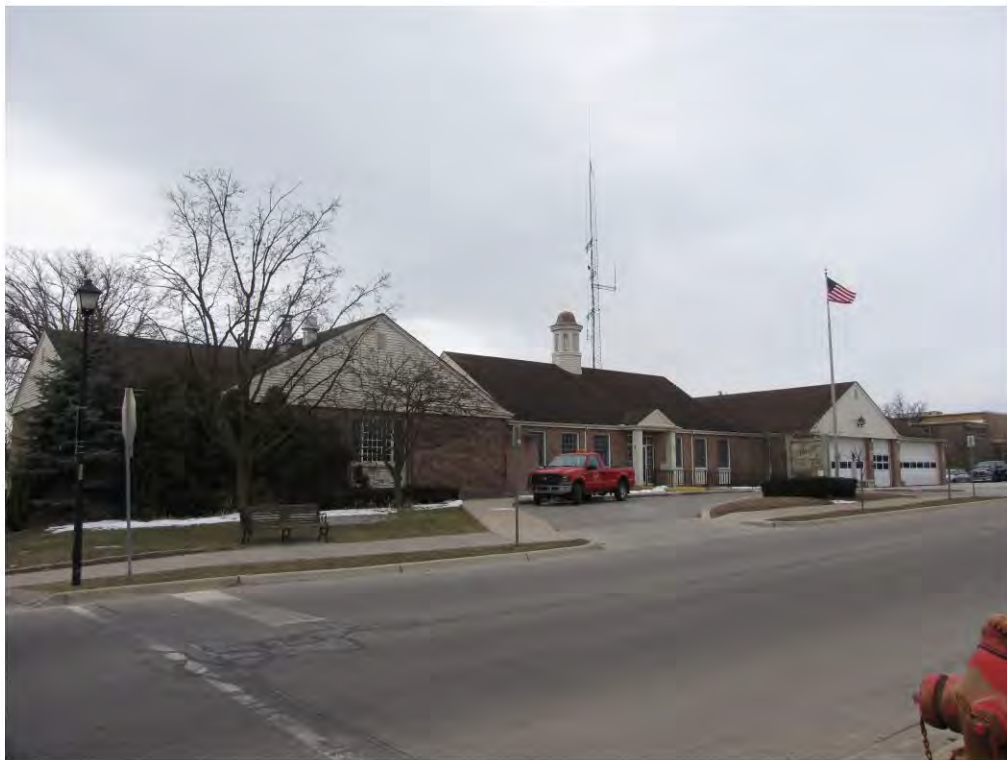
Main West 215_Looking Southwest
