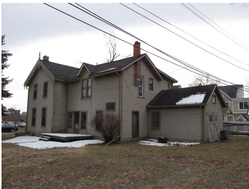
Wing North 129_Looking Southeast
