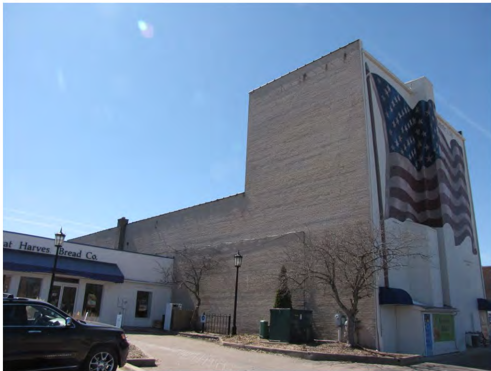
Main East 135-137_Looking Southwest
