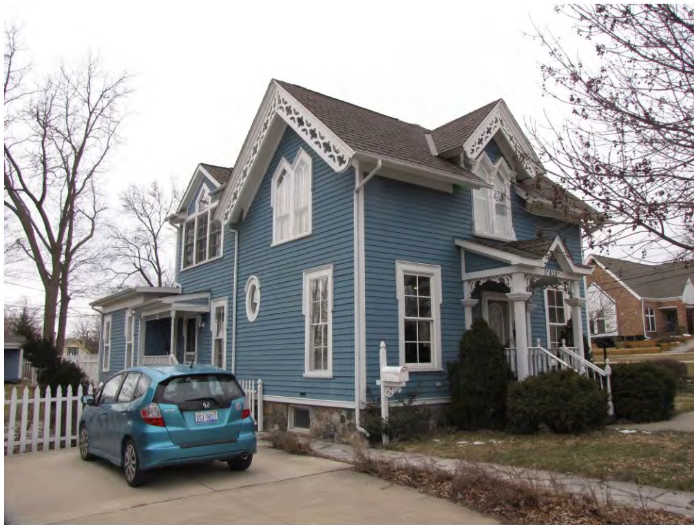
Main East 410_Looking Southwest
