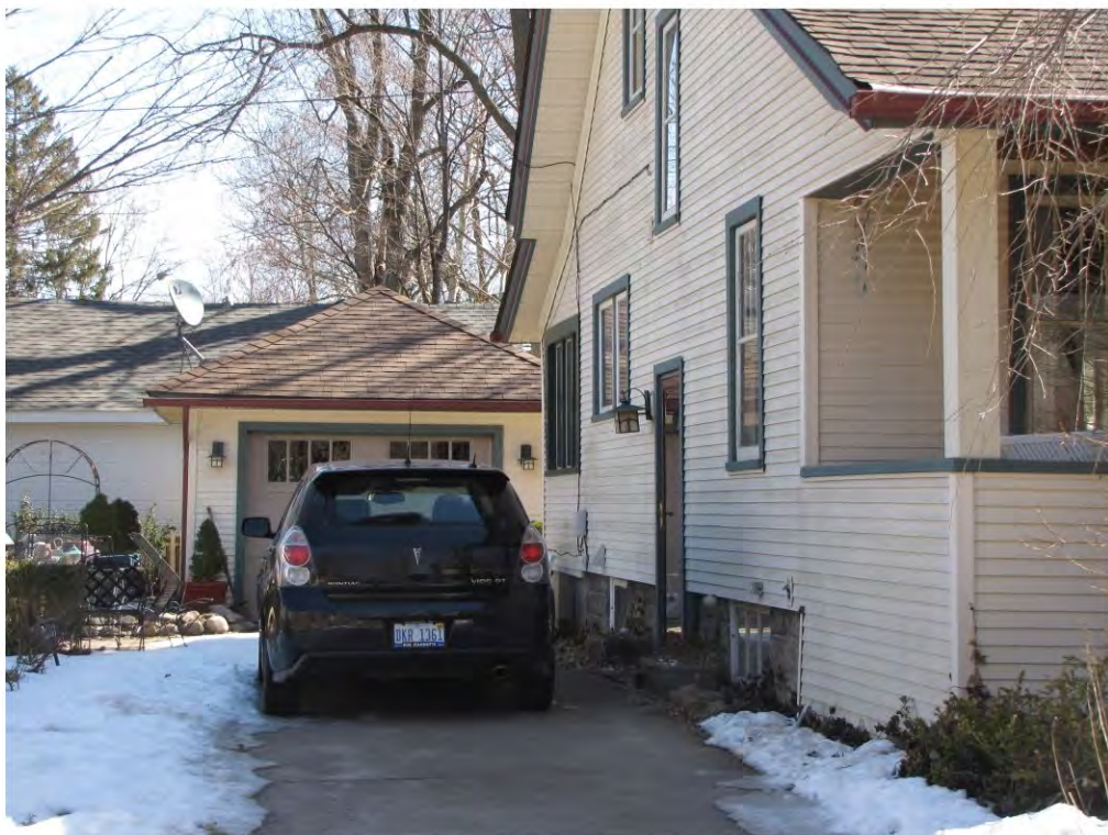
Linden 118, Garage_Looking East
