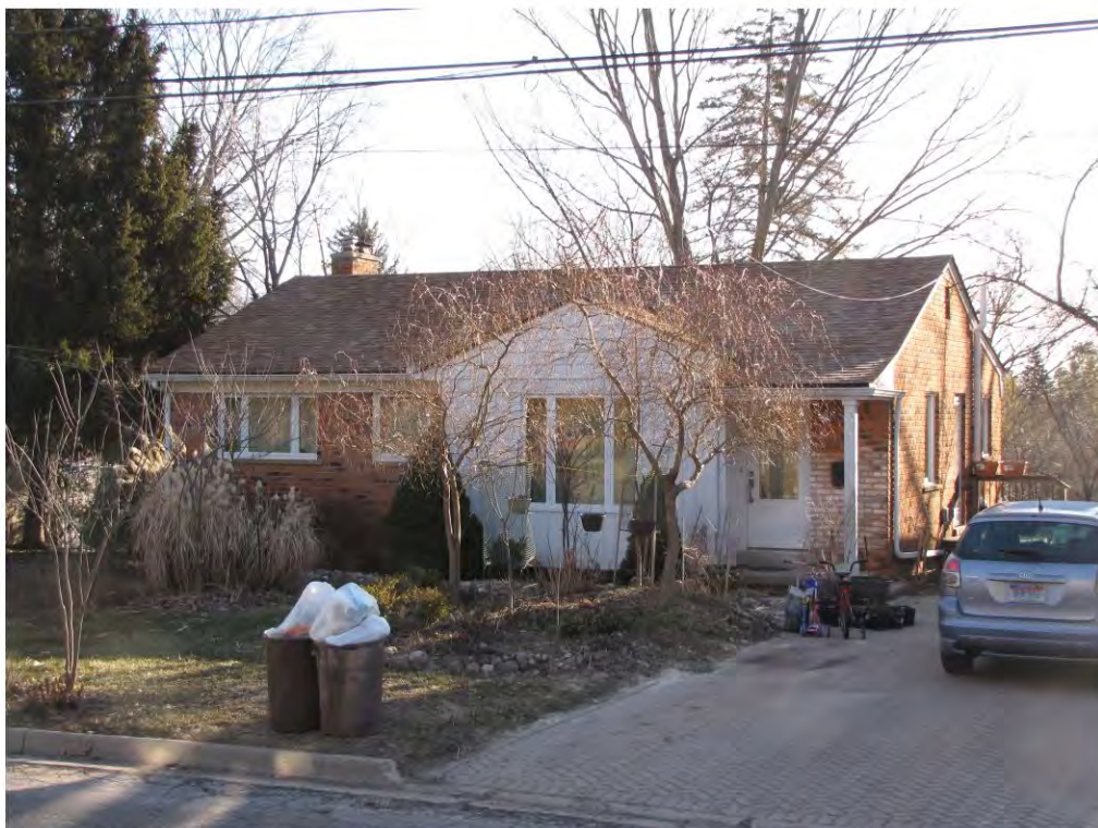
Rogers North 368_Looking Northeast
