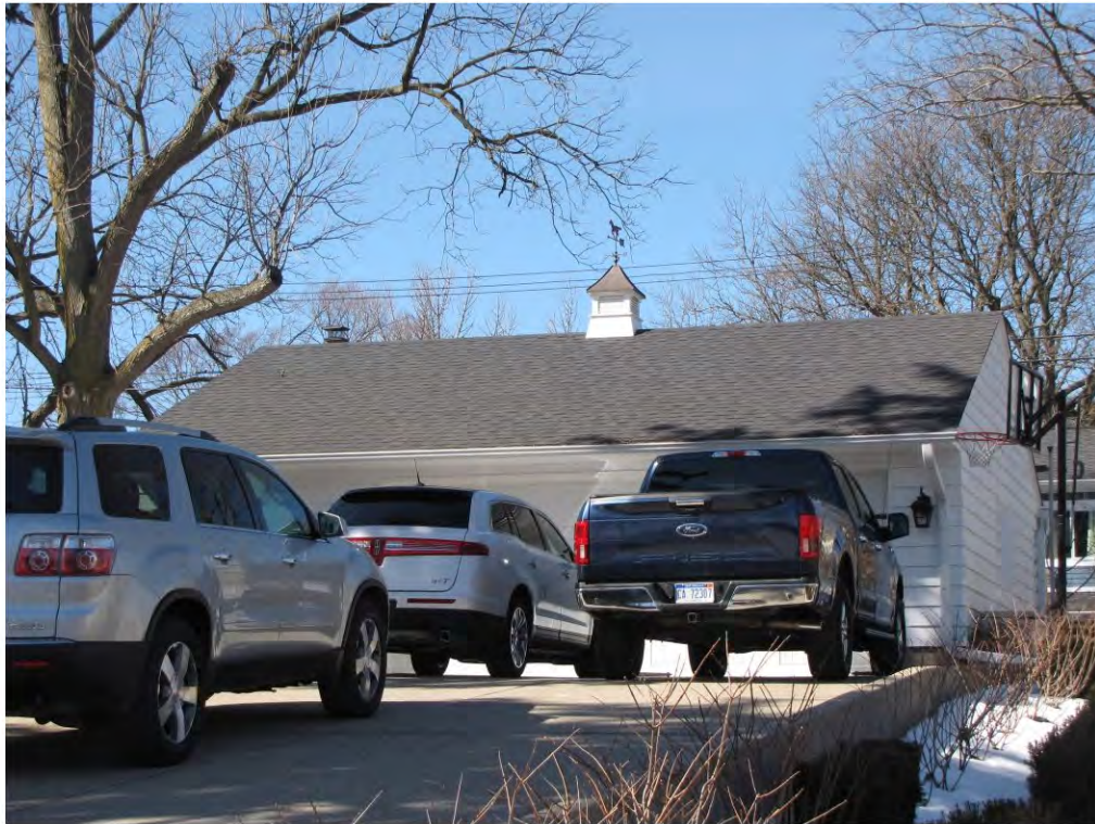
West 247, Garage_Looking West
