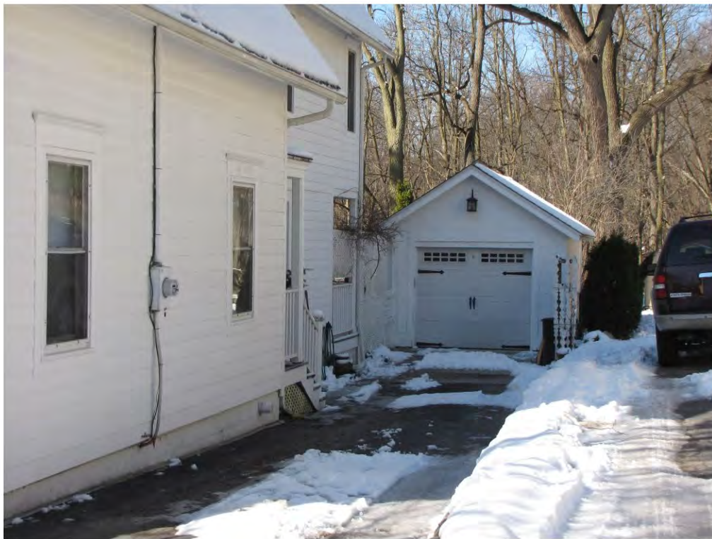
Rogers North 207, Garage_Looking West
