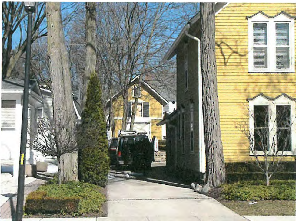
Main West 536, Garage_Looking N011h
